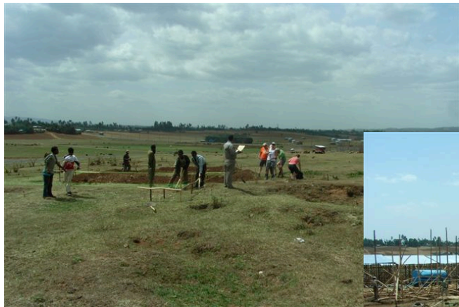
The building site for 45 houses
